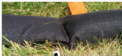
Overlap Flap: No gapping at connections
